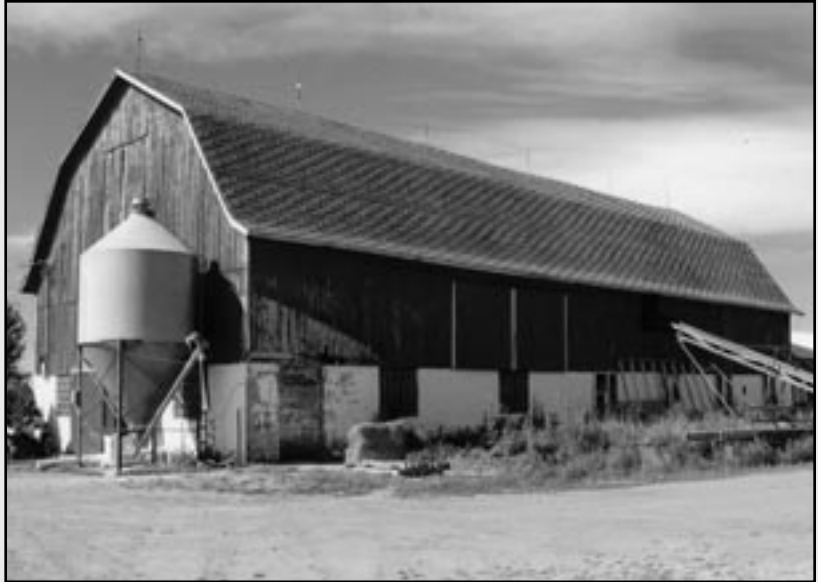
An old dairy barn is home to chicks for the first four weeks until they are ready to go out on pasture.
